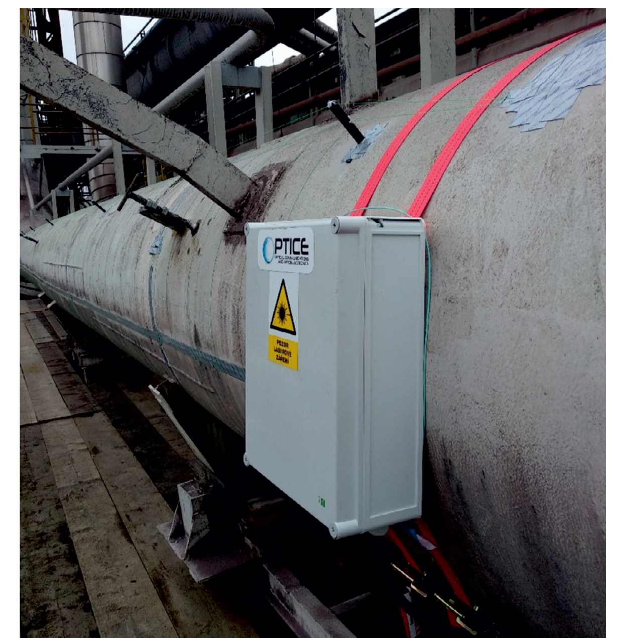
Obr. 1: Real measuring location
